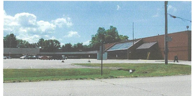
Underutilized Shopping Center Along Morton Ave.
